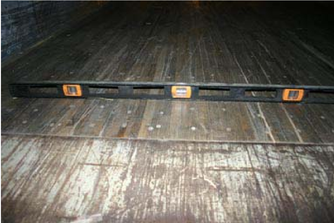
Flatness of composite flooring at a forward section.
