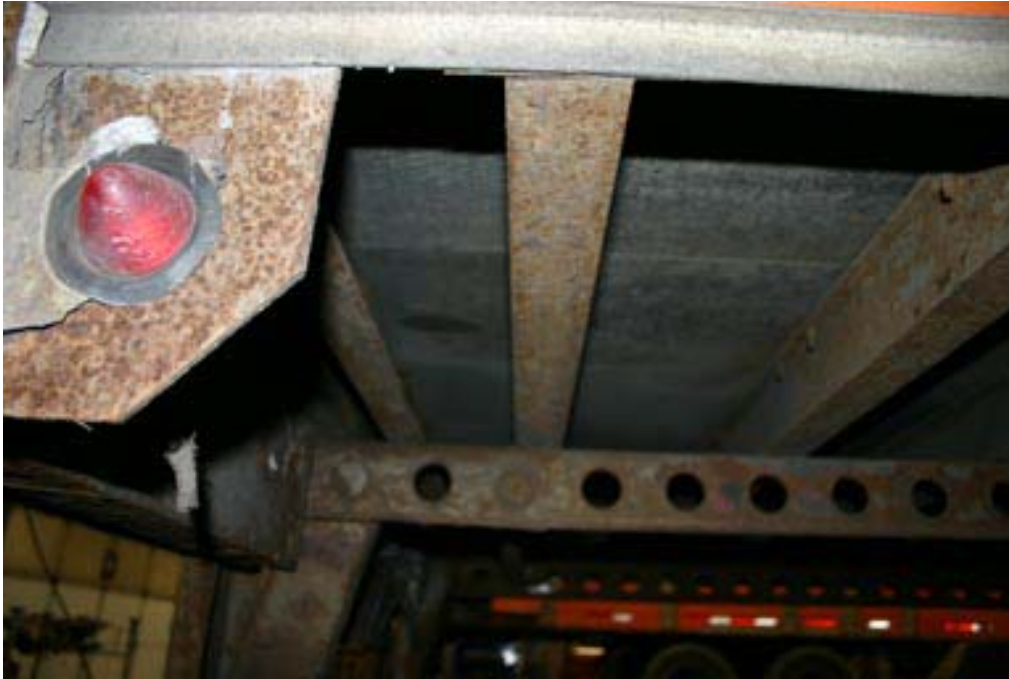
Underside of composite flooring at the rear section.
