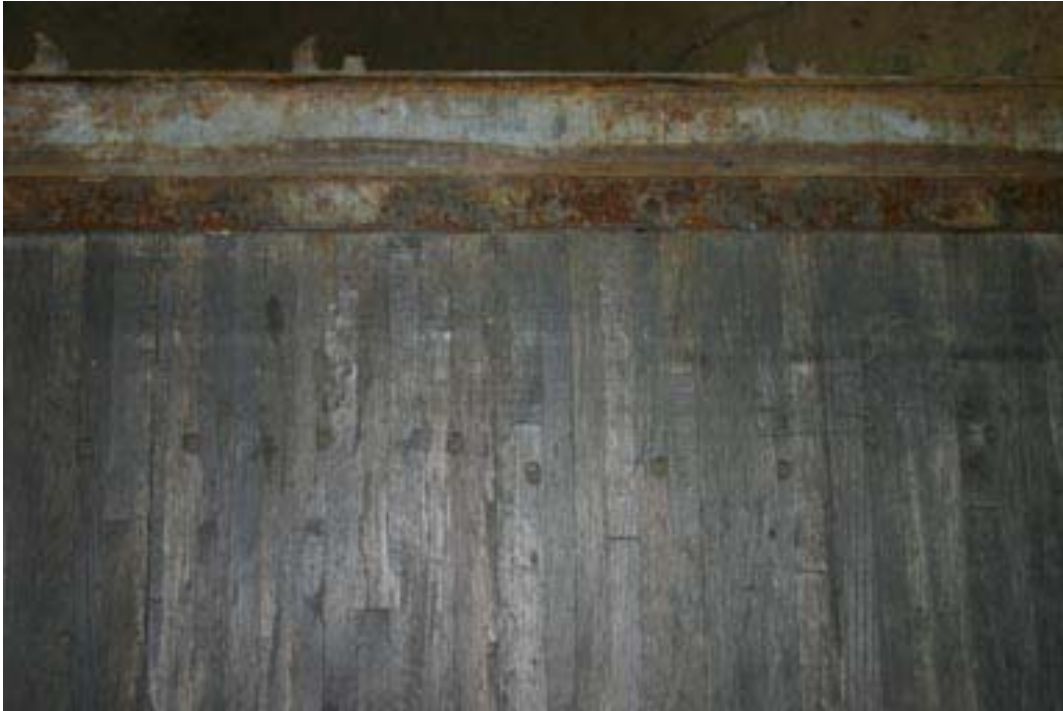
Top side of rear section of composite flooring.
