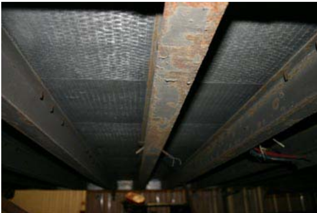
Underside of composite flooring in the bay section.
