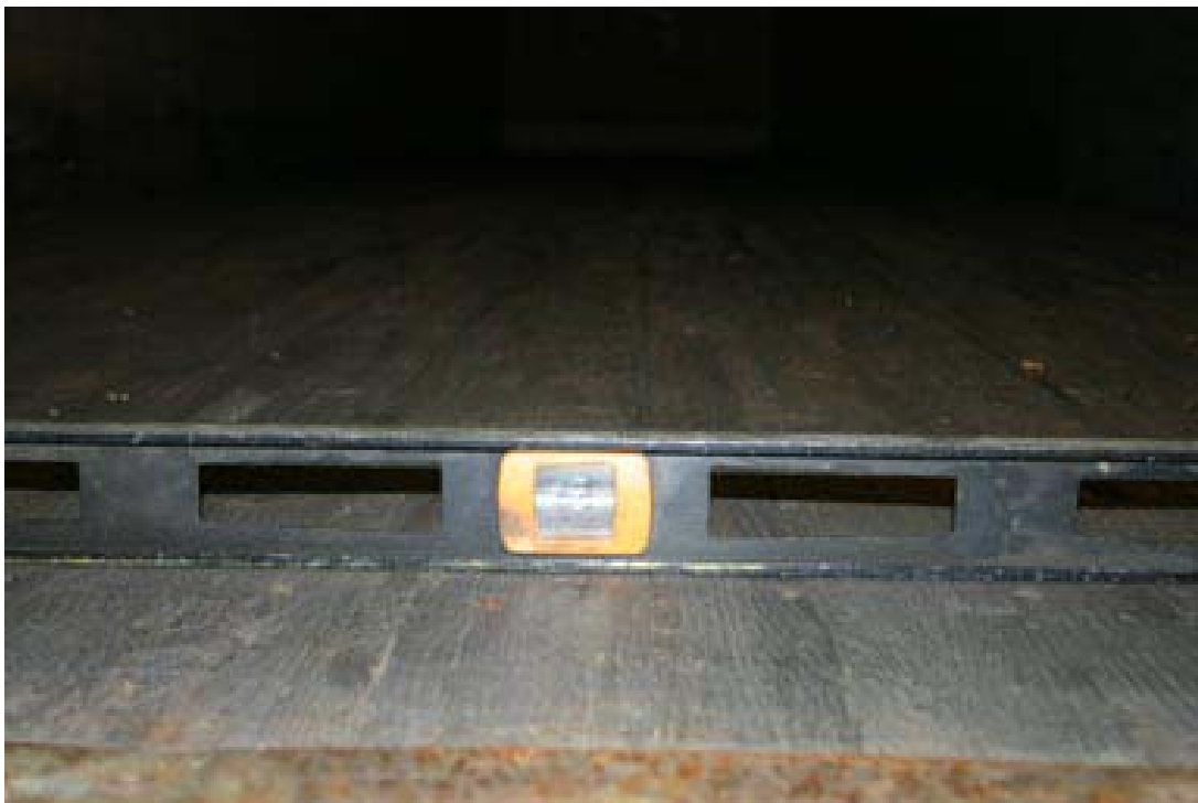
Flatness of composite flooring at a rear section.
