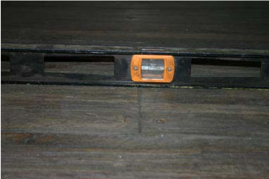
Flatness of composite flooring across a butt joint of boards.
